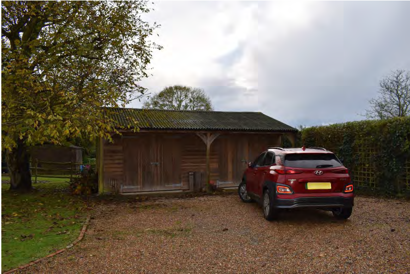
Plate 15: View of the garage (facing S)
